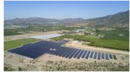
The large-scale solar PV power plant in El Boco, Chile, is the second project of BELECTRIC's PMGD project portfolio
