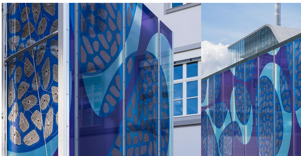
OPV modules, integrated in colour-printed, translucent ETFE films.
